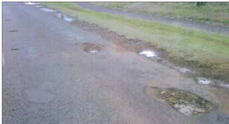
Highfields Road - More than 50 potholes repaired after rain.
